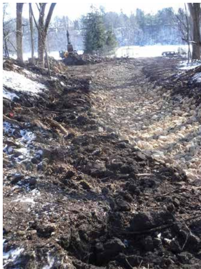
Outlet of ravine after construction completed. Courtesy of Dunn County.
